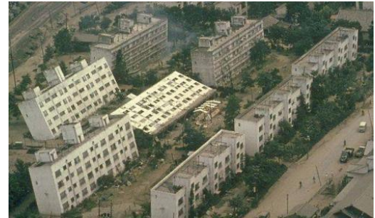
Figure 2. liquefaction damage caused by the 1964 Niigata Earthquake
